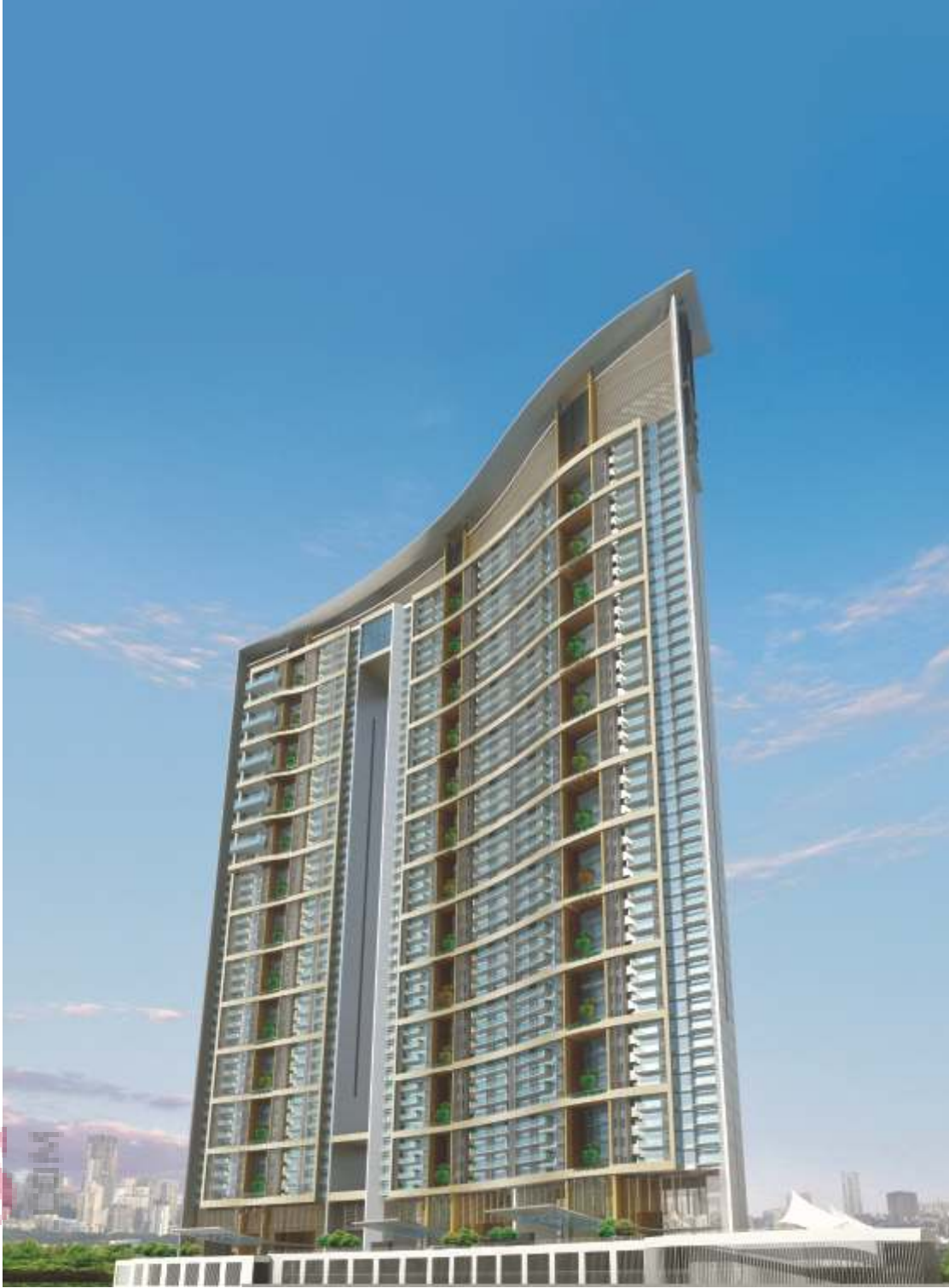
West side façade
