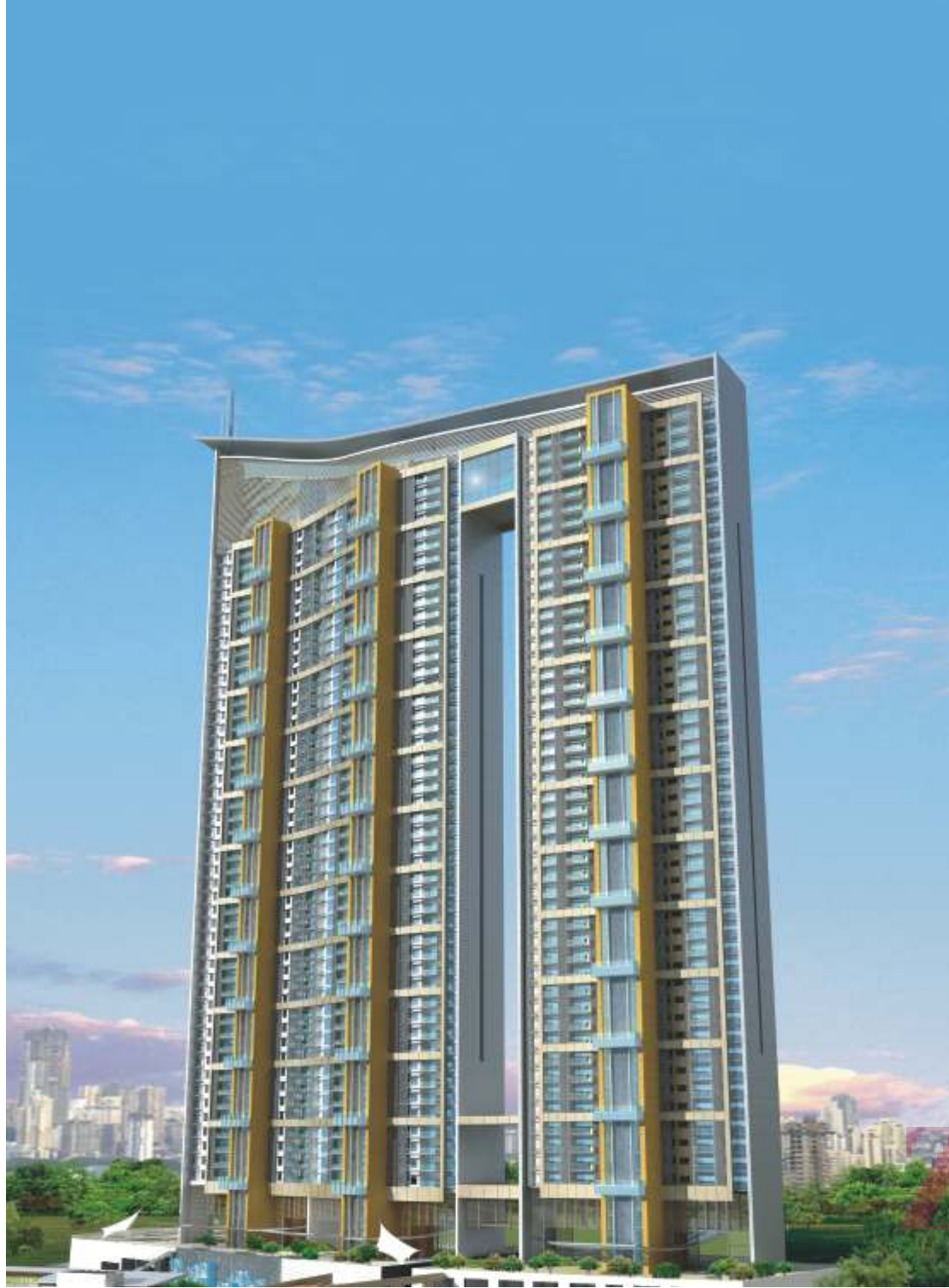
East side façade
