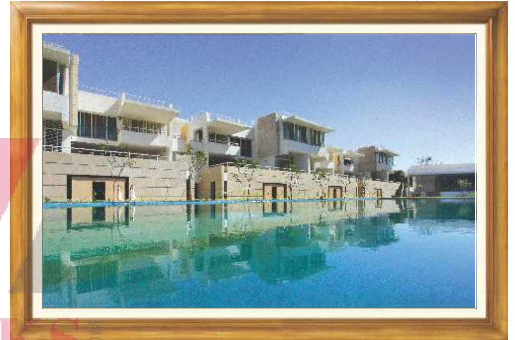
ROHAN MADHUBAN, BAVDHAN, PUNE
