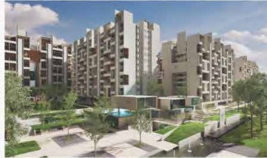
Rohan Abhilasha, Lohegaon-Wagholi Road, 7 Km from Pune Airport
