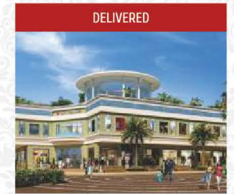
CITY SQUARE Commercial Complex at ACE City Sec-01, Gr. Noida (West)
