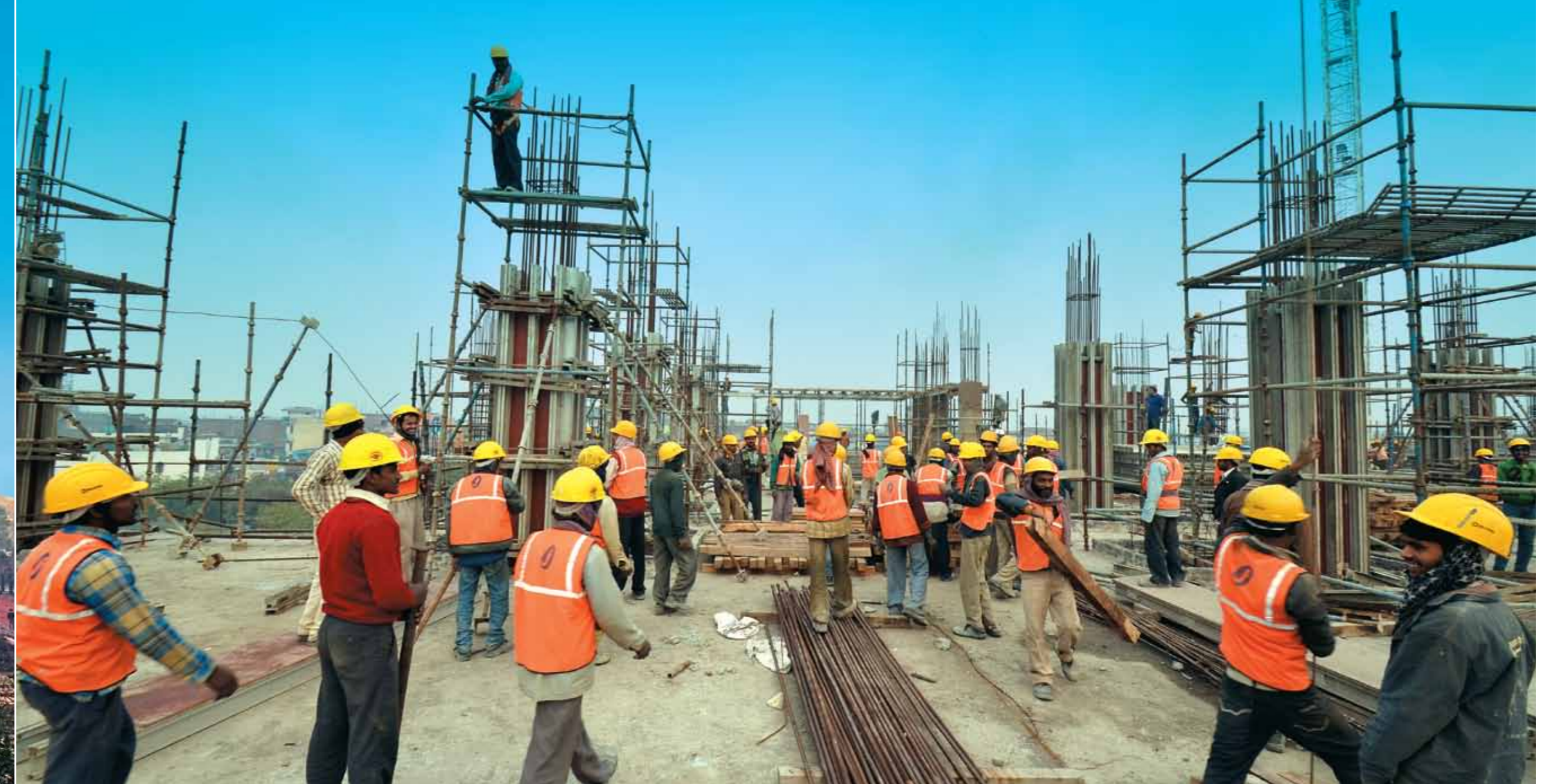
Actual site image as on 31-01-2013
