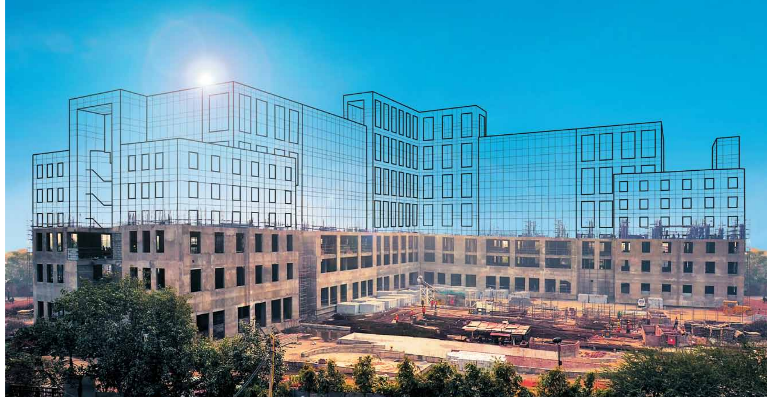
Actual site image as on 31-01-2013
