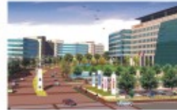
DLF Atrium IT SEZ @ Pune**
