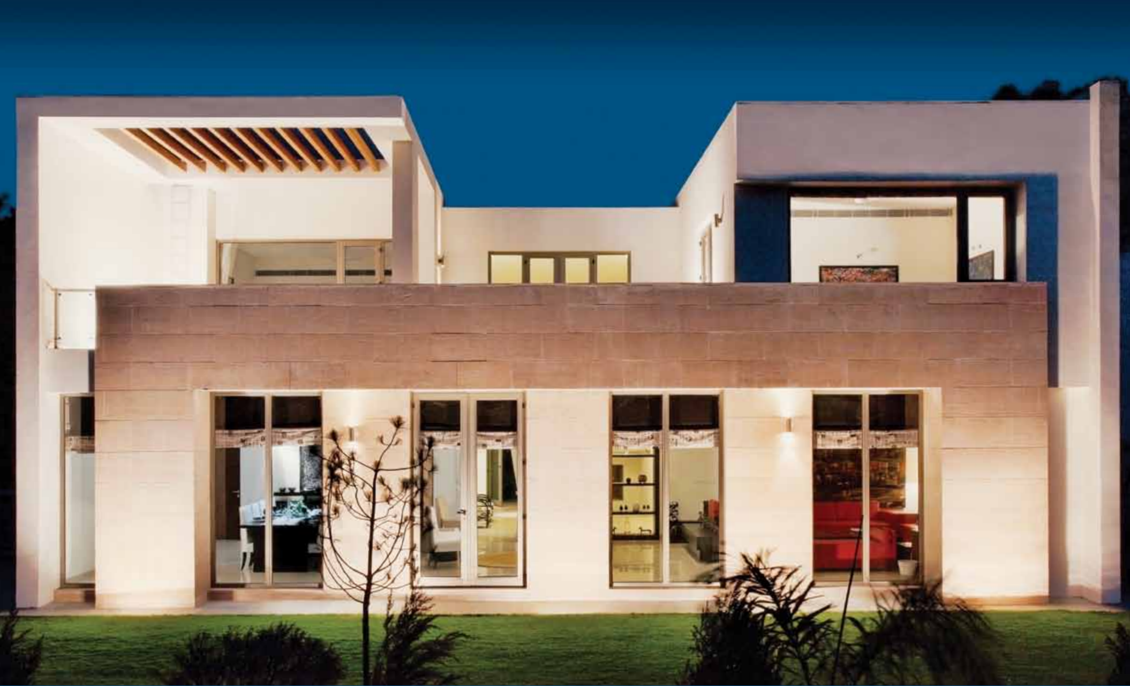
100% power back up
