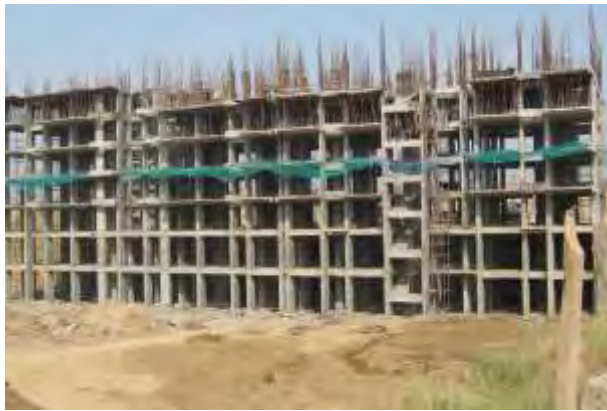
Navodaya - construction photograph
