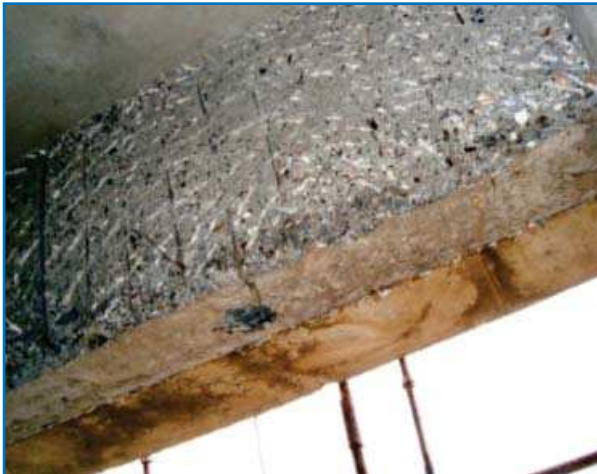
Chipping of beam (Report No. 9-Tower 1)
