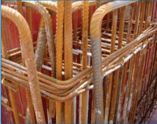
Main bars of the beams located outside the vertical bars of the column - Report No. 3
