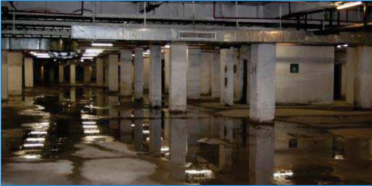
Photograph of the basement taken by audit in January 2011
