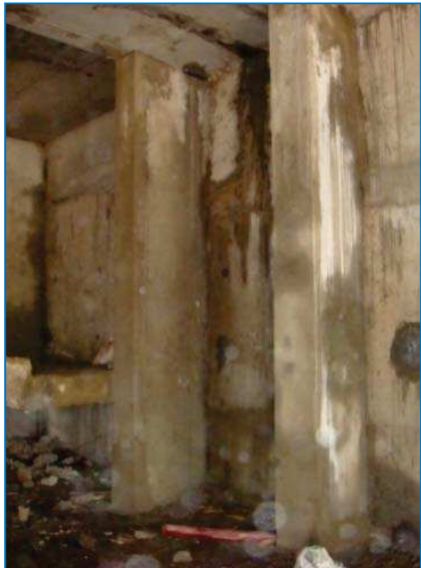
Another column in Tower-5 after cosmetic treatment (Report No. 3)
