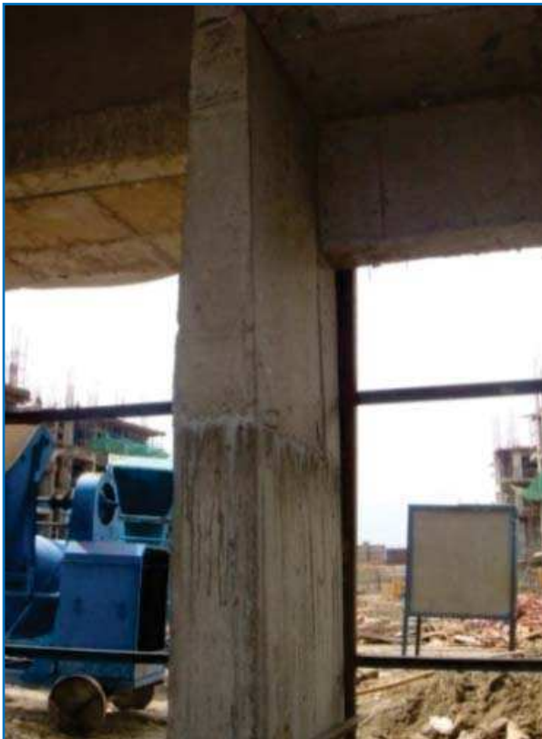
Tapered Column in the Basement of Tower-3 (Report No. 3)
