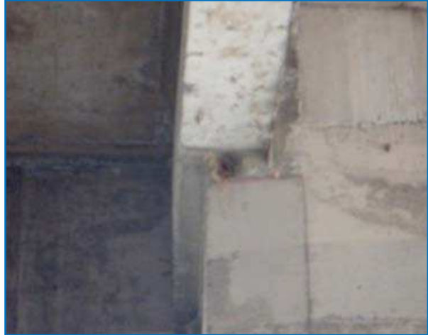
Half the width of the beam is outside the column - Report No. 3
