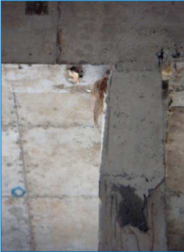
Tapered and Bent up Column in the Basement of Tower-3 (Report No. 3)
