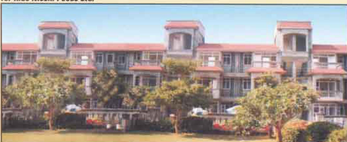
Olive Apartments, at Sushant Lok- II
