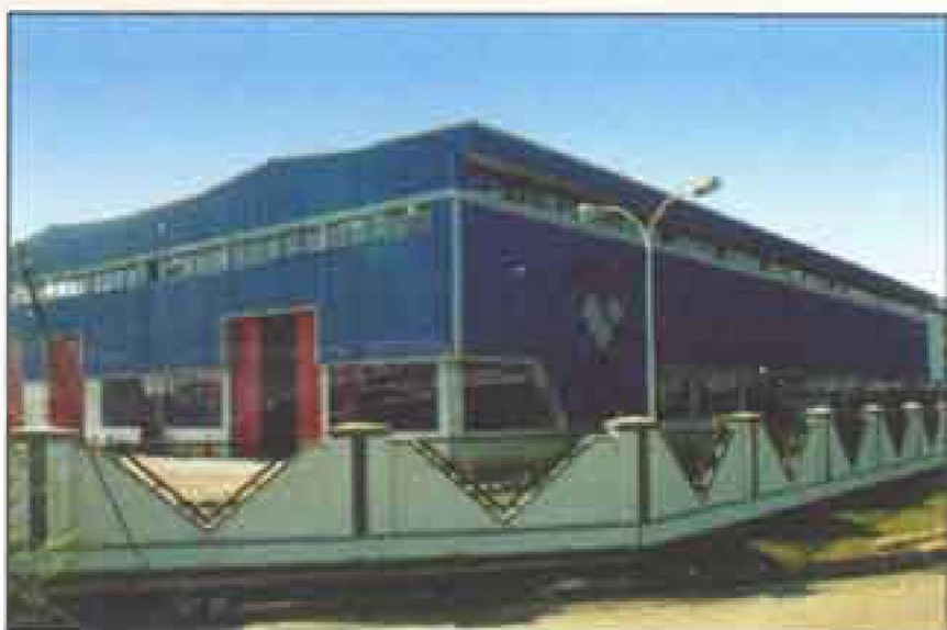
Mfg. Plant, at Gurgaon for Swedala Industri India Pvt. Ltd.
