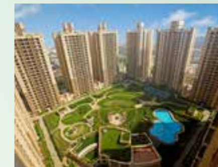
ATS ADVANTAGE PHASE I Indrapuram
