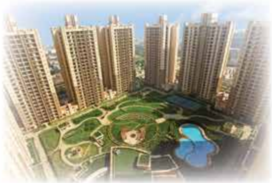
ATS ADVANTAGE PHASE I Indrapuram
