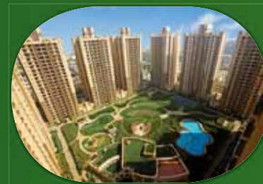
ATS ADVANTAGE PHASE I Indrapuram
