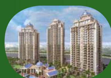
ATS MARIGOLD Gurgaon
