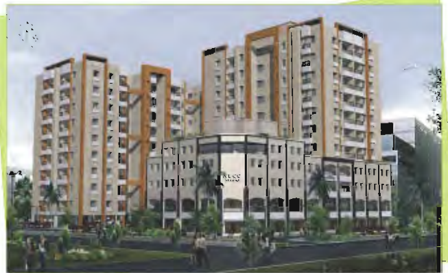
NBCC Tower - Patna
