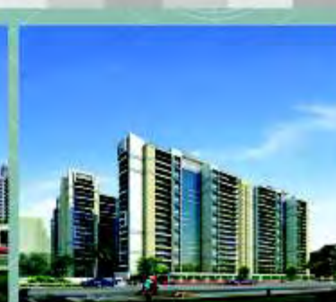
Ongoing Prateek Stylome Sector-45, Noida
