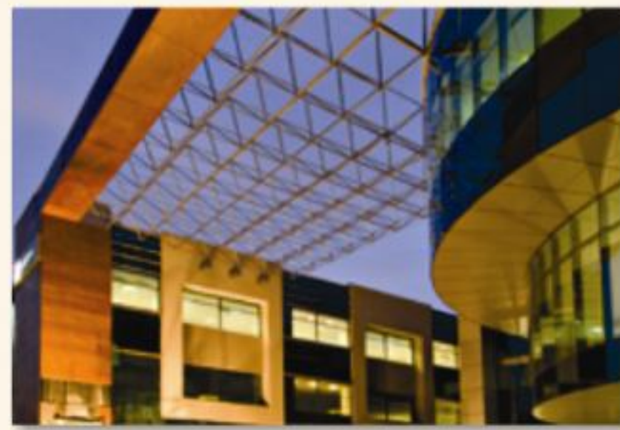
PATNI KNOWLEDGE CENTER, NOIDA (BLOCK B) GOLD RATED LEED CERTIFIED GREEN BUILDING - 2011
