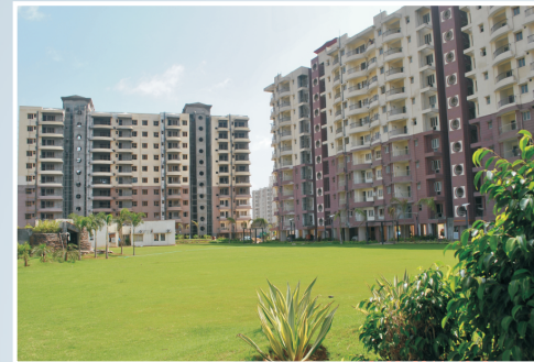
Actual Site Photograph of Krish Vatika
