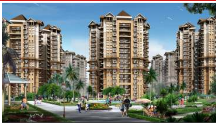
SRS RESIDENCY, SECTOR - 88, FARIDABAD (Construction In Full Swing)
