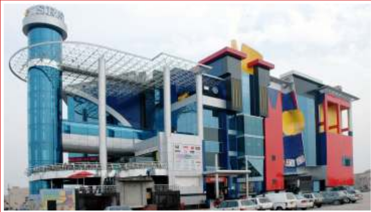
SRS MULTIPLEX, CITY CENTER, SECTOR - 12, FARIDABAD (Successfully Running)
