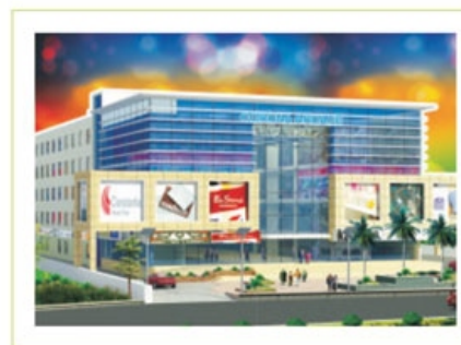
CORONA ARCADE NH-10 BAHADURGARH
