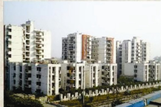
EASTEND APARTMENTS (INDIRAPURAM)
