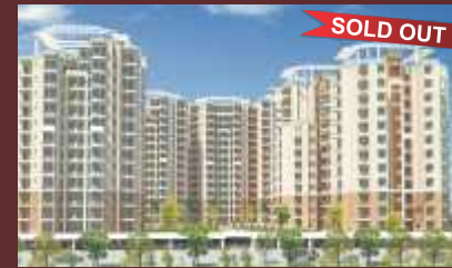
KLJ HEIGHTS, Sector 15, Bahadurgarh
