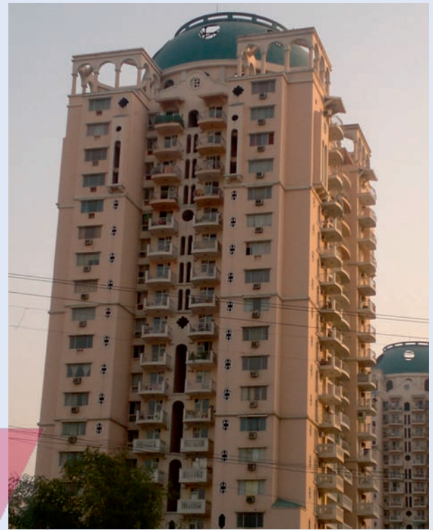
DLF Trinity Tower, Gurgaon
