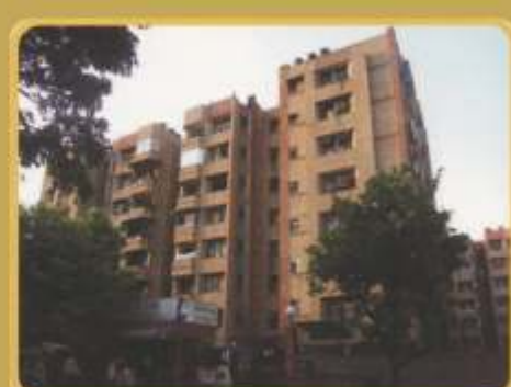
DSIDC Co-operative Apartments Plot 23, Sec - 9, Rohini Delhi Consisting 135 units
