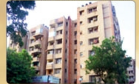
DSIDC Apartments Plot 23, Sector 9, Rohini, Delhi
