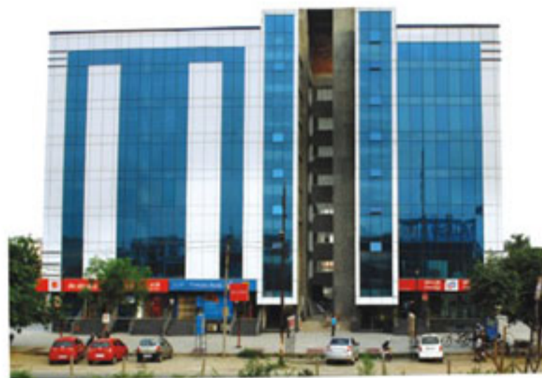
SG Alpha Tower-1, Vasundhara (Ready for possession)
