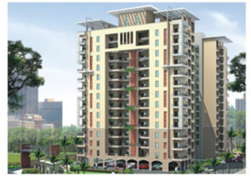
ImpressionsPlus, Rajnagar Extn., Ghaziabad (Under Construction)
