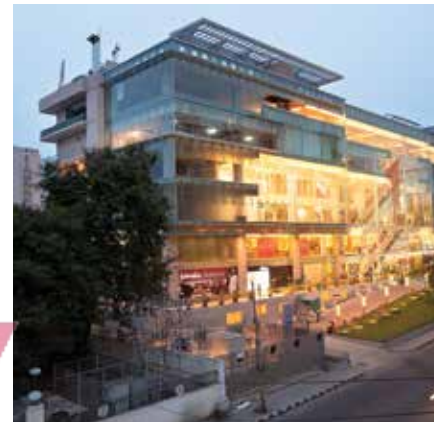
1 MG ROAD MALL Bengaluru
