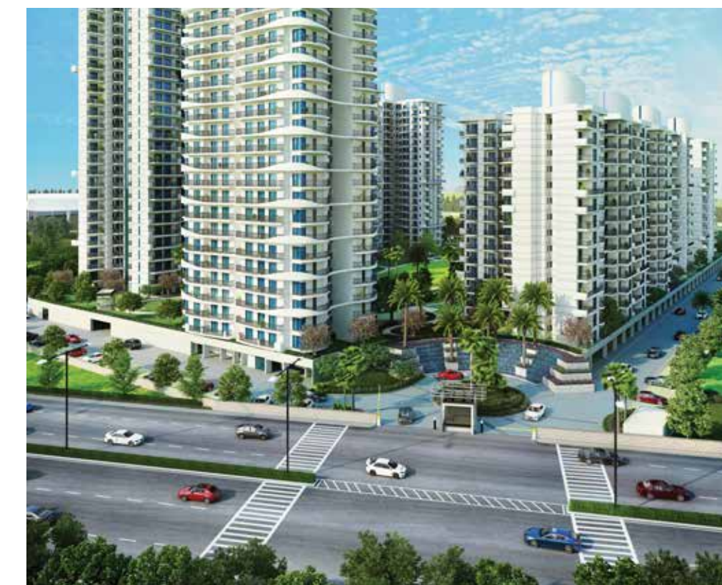
The project is situated on the 30 m wide sector road which is connected to the Gurgaon-Sohna State Highway.
