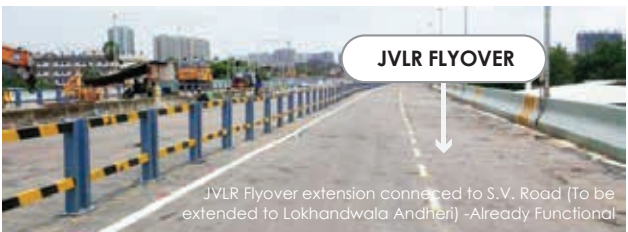
Six 90 feet road under construction to connect ODC to S.V. Road
