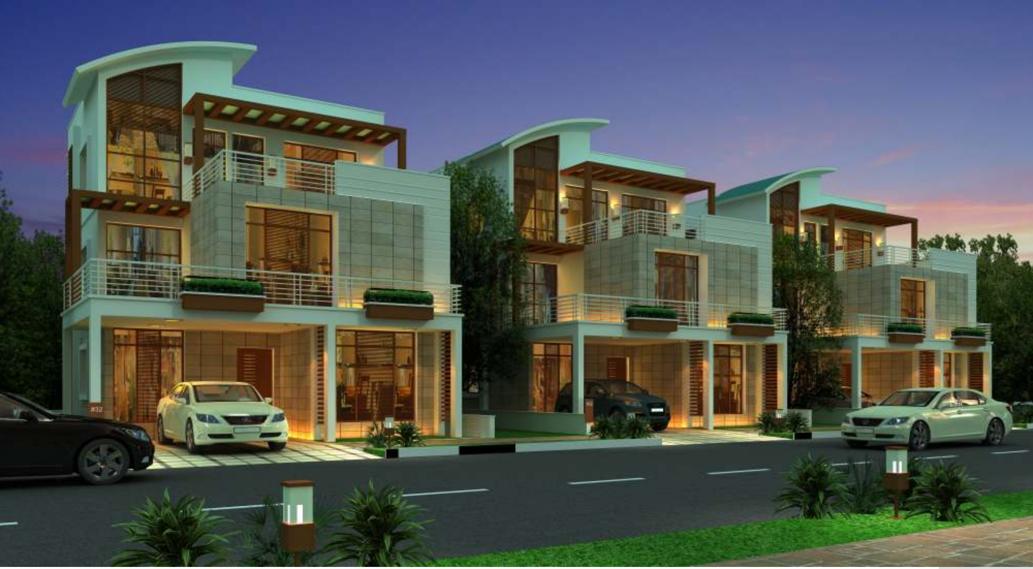
North facing street view
