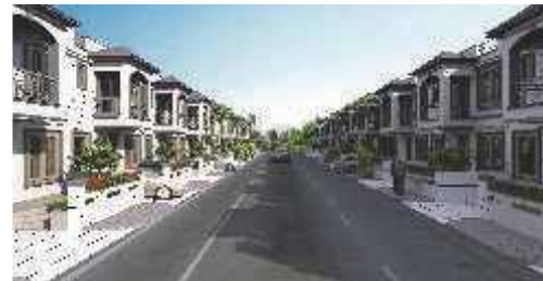
Prime Ville (90-Villas) Mahapura, Ajmer Road, Jaipur
