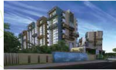
EASTCREST Near Budigere Cross, Bangalore
