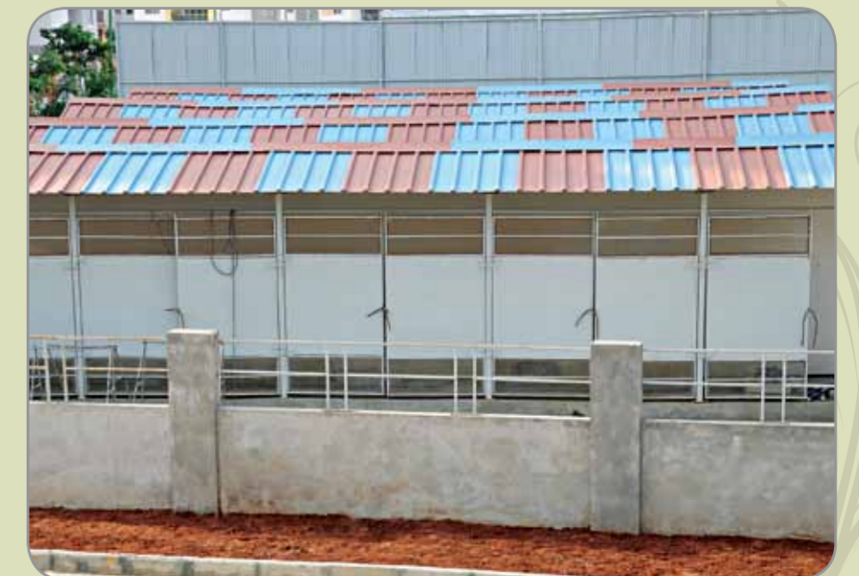
Piped Gas Storage Center
