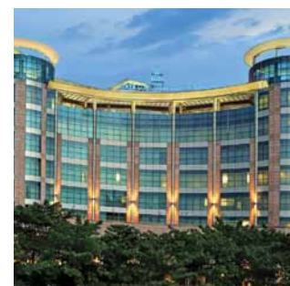
SHALIMAR TCS BUILDING
