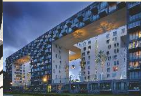
Parkrand Building, Amsterdam
