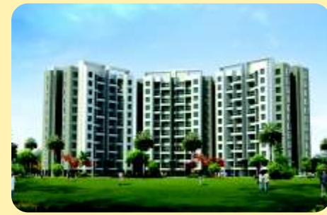
GULMOHAR QUEENSTOWN Kharadi
