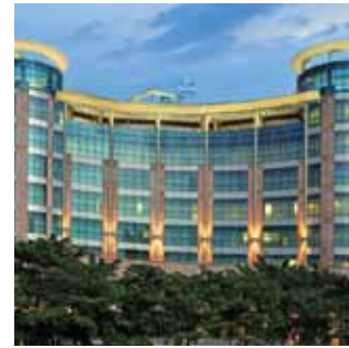
SHALIMAR TCS BUILDING
