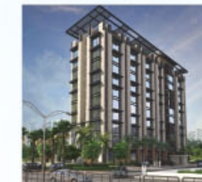
AKSHAT RETREAT at Opp. SMS Hospital Jaipur's First Ever LEED Compliant Commercial Building entirely dedicated to healthcare
