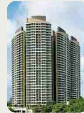
KALPATARU TOWERS KANDIVALI
