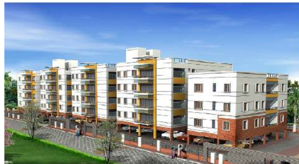
BOLLINENI HILLSIDE, ONGOING RESIDENTIAL TOWNSHIP AT OMR, CHENNAI
