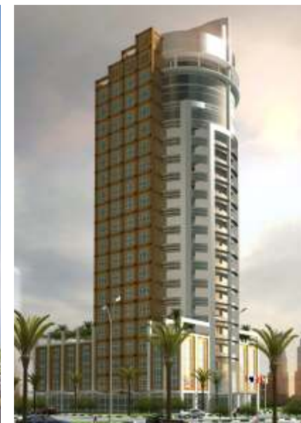
JUMERA VILLAGE, ONGOING HOTEL PROJECT, DUBAI
