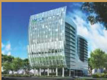
IT Twin Tower Sector 66-A
