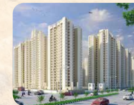
ATS ADVANTAGE PHASE II Indirapuram
