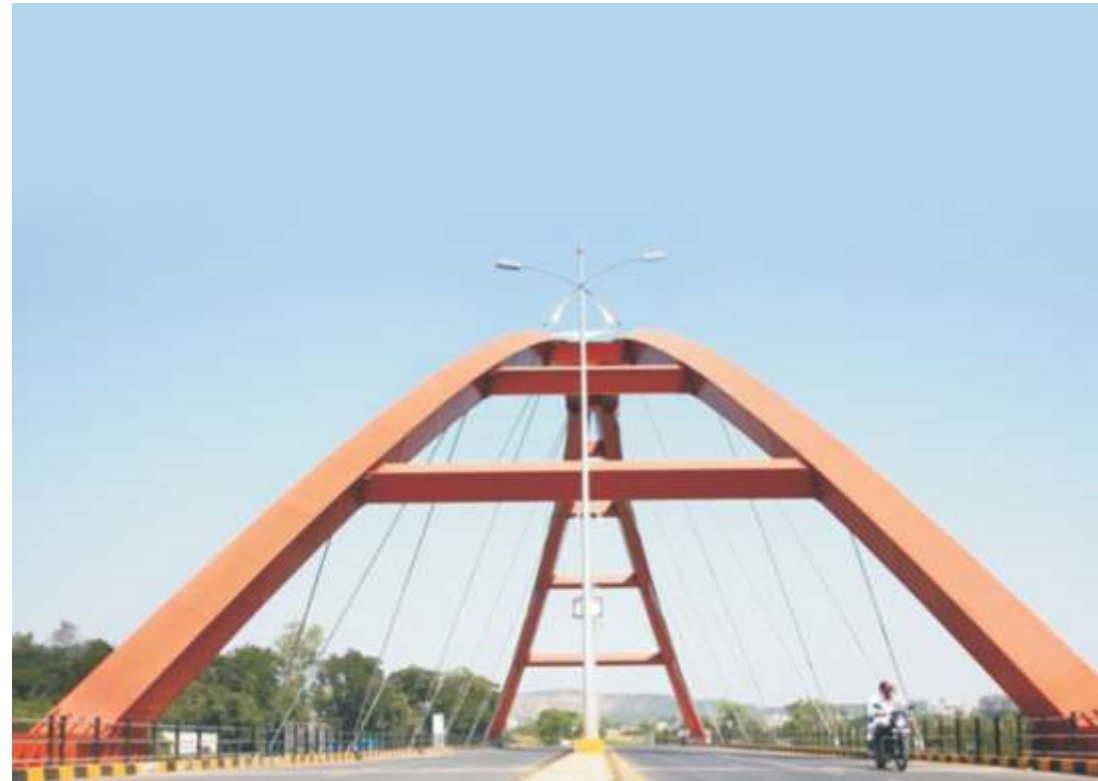
Basket Bridge, Ravet
