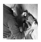
Electrical conduits cut by a machine and debris scooped out by a scooper instead of using a hammer and chisel to reduce stress on bricks and avoid cracks
