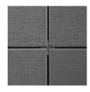
Spacers used for wall tiles to ensure correct alignment of tiles and to improve aesthetics
