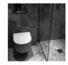
Toilets strictly designed to divide dry and wet areas. Shower area provided with a step down of 1/2" inch to avoid water spilling over to the dry area
