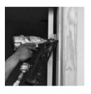
Door frames drilled and anchor bolted to the brick wall to provide better strength and durability
