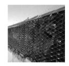
Electrical conduits covered with a mesh before plastering with cement plaster mixed with Recron to avoid cracks
