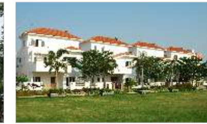
Residential villas, at Hyderabad
