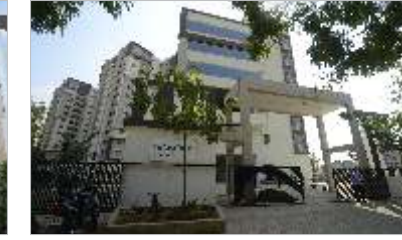
High-rise apartments, Tellapur
