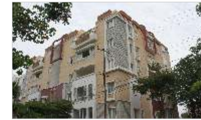
Residential towers at Madhapur
