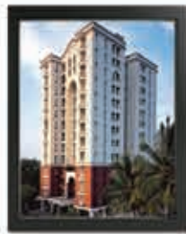
MARBLE ARCH Kaloor
