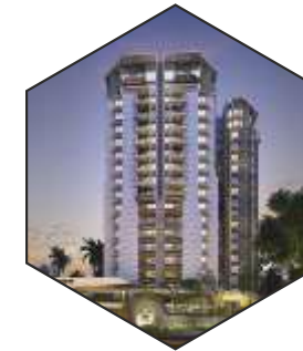
OASIS Unichira, Edappally
