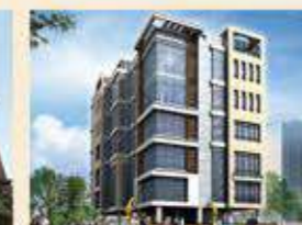
Commercial at EM Bypass
