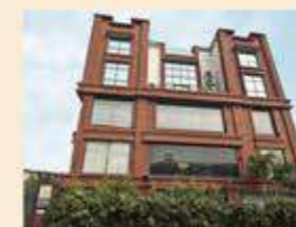
Commercial at EM Bypass
