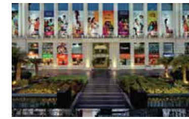
SHALIMAR ELLDEE PLAZA, BHOOTNATH MARKET, LUCKNOW
