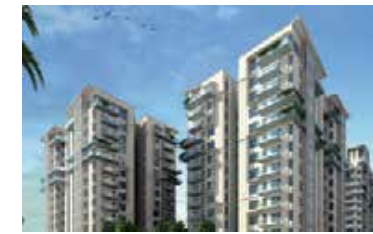
SHALIMAR GALLANT, MAHANAGAR, LUCKNOW UPRERAPRJ3168
