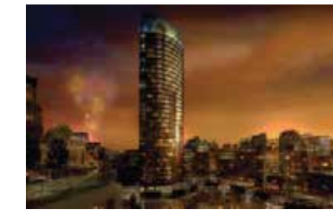
SHALIMAR ONE WORLD, GOMTI NAGAR EXTENSION, LUCKNOW UPRERAPRM10813
