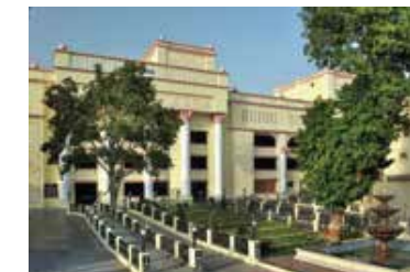
MULTILEVEL PARKING, HAZRATGANJ, LUCKNOW
