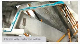
Water channels to collect construction water and rain 100% non-porous walls + Highly seismic-resistant
